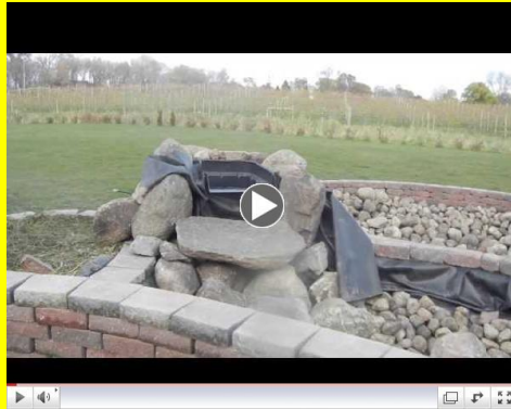
Pond waterfall construction.
